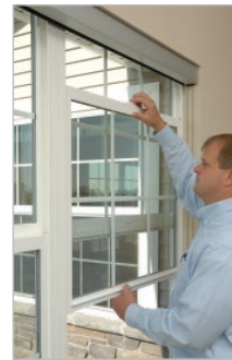
3. Shift sash to right within channel
